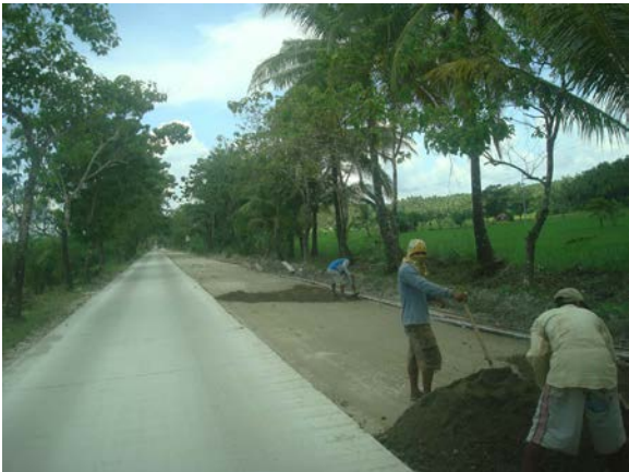
a. Manual laying out of sub-base material
