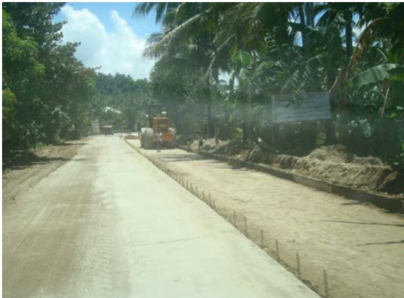
b. Compaction of sub-base layer
