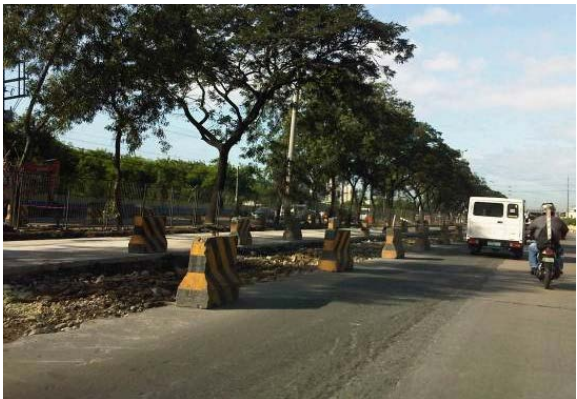
a. Rehabilitation along urban highway
