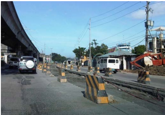
b. Typical road works along urban highway
