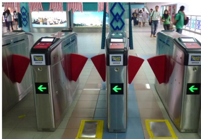
Figure 1. Example of automatic ticketing gates at Malaysian rail transit station
