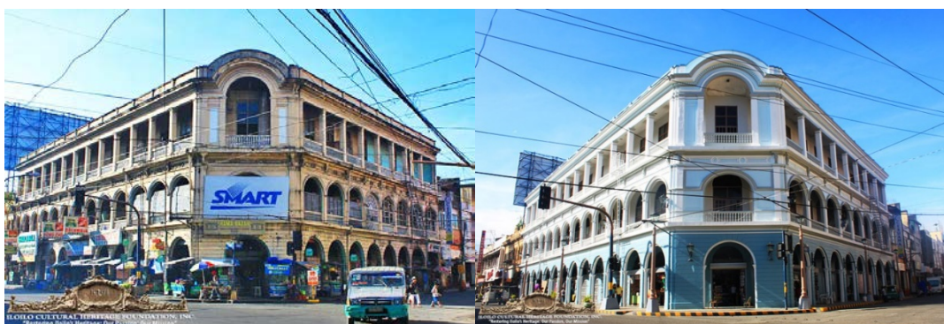
Figure 3. A heritage building before (left) and after restoration (right)
