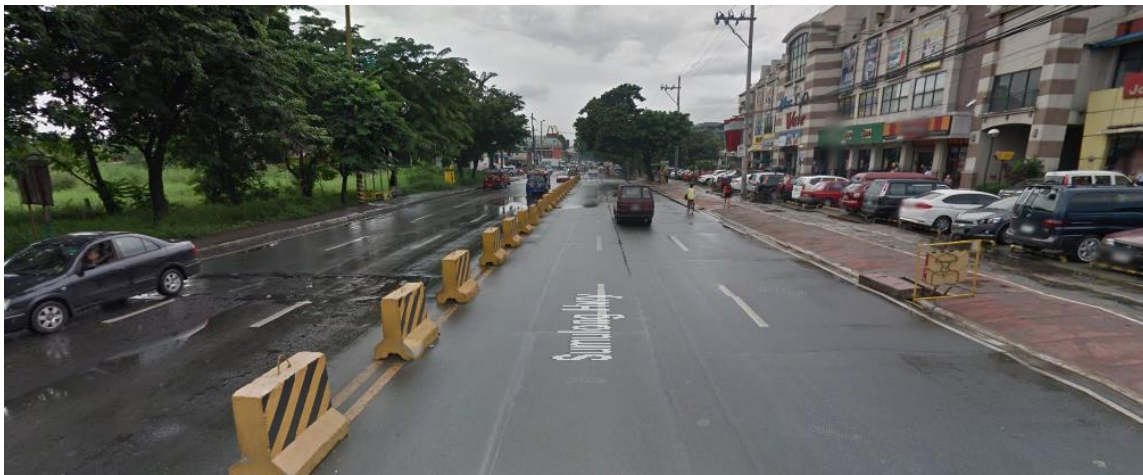
Existing Sumulong Highway in Marikina
