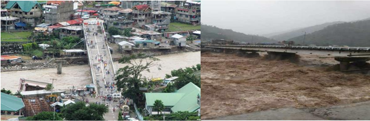
Figure 9. The connecting bridge from Bontoc, going to Banaue was displaced thus visitors and locals need to walk the bridge since heavy vehicles are not allowed to traverse the bridge after being displaced by the typhoon (Source: Google.com)
