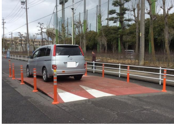
Figure 15. View of trial installation of portable humps
