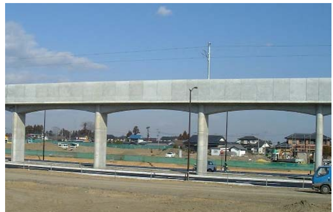
Photo 11: The arch slab-type elevated track that considered as landscape
