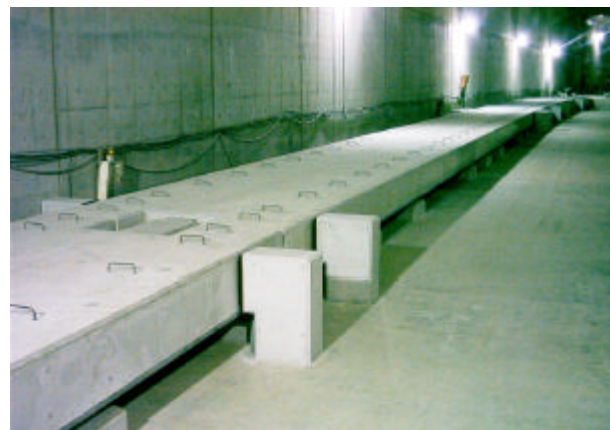
Photo 5: The floating slab
