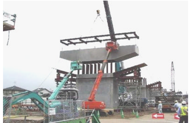
Photo5: Prefabricated composite substructure
