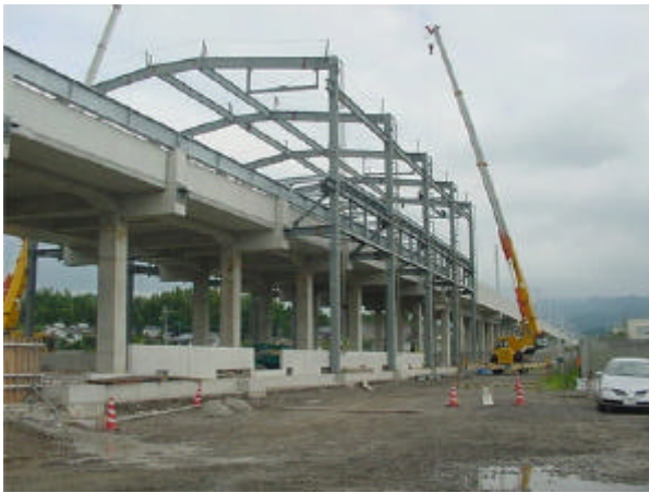
Photo 7: Station construction by Architecture
