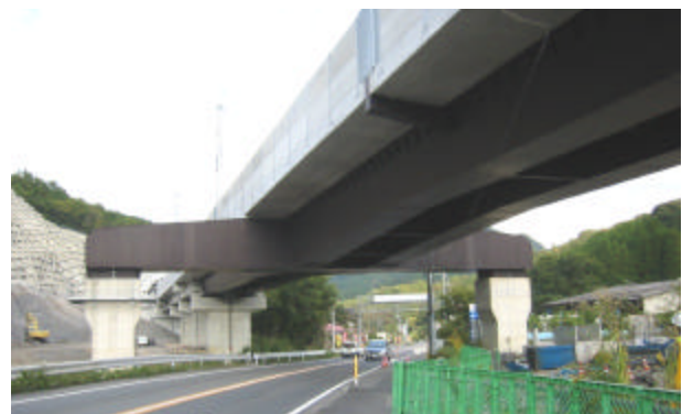
Photo6: Portal frame subgirder
