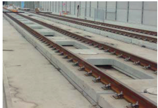
Photo8: Frame type concrete slab track
