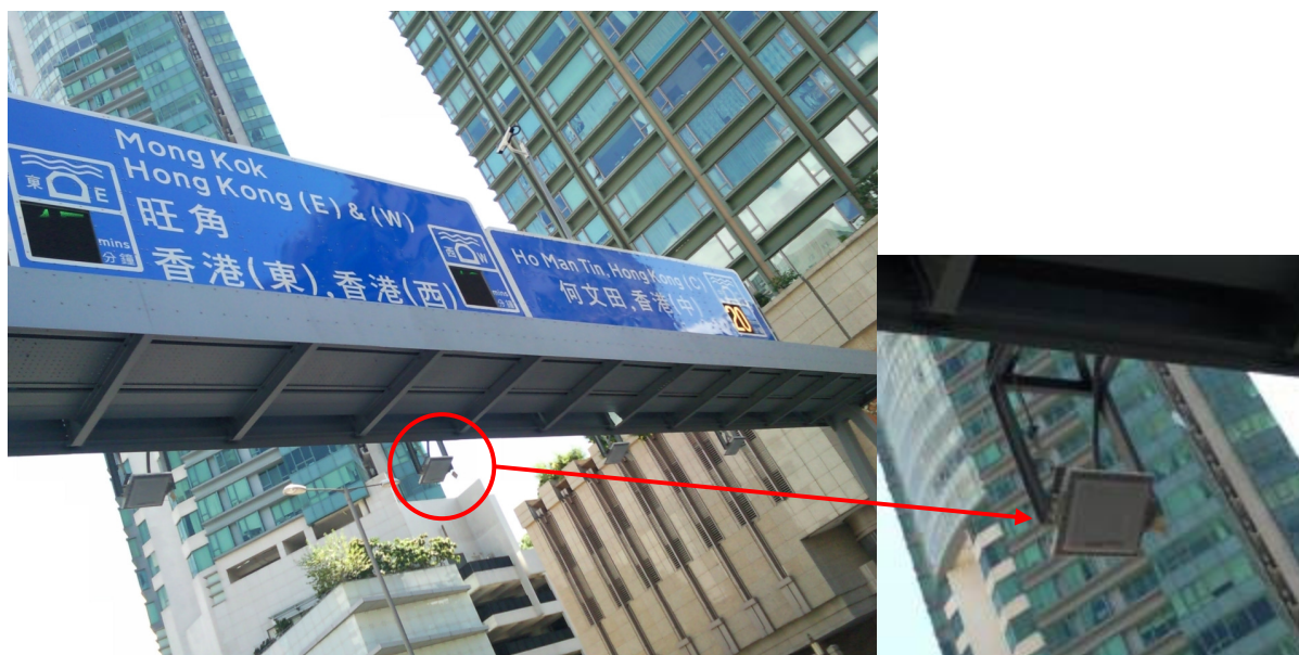
Figure 3. AVI Tag Readers Installed on Gantry
