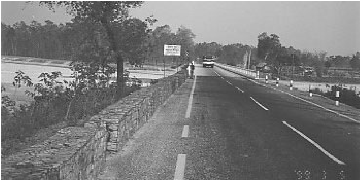
Figure 2. Use of SFWC barrier on high embankment
